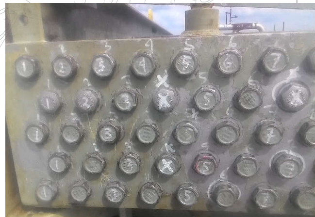
Result Leak Test Header Box
