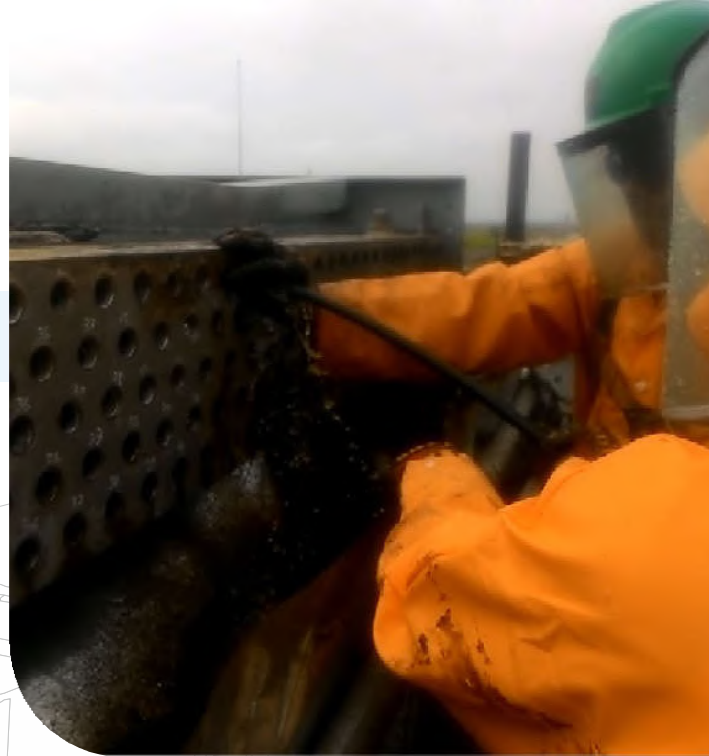
Mechanical Cleaning with Flexible Lance
