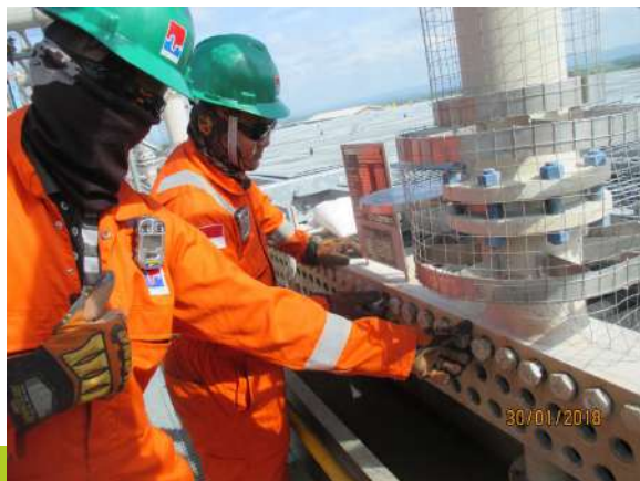
Inspection of Header Box
