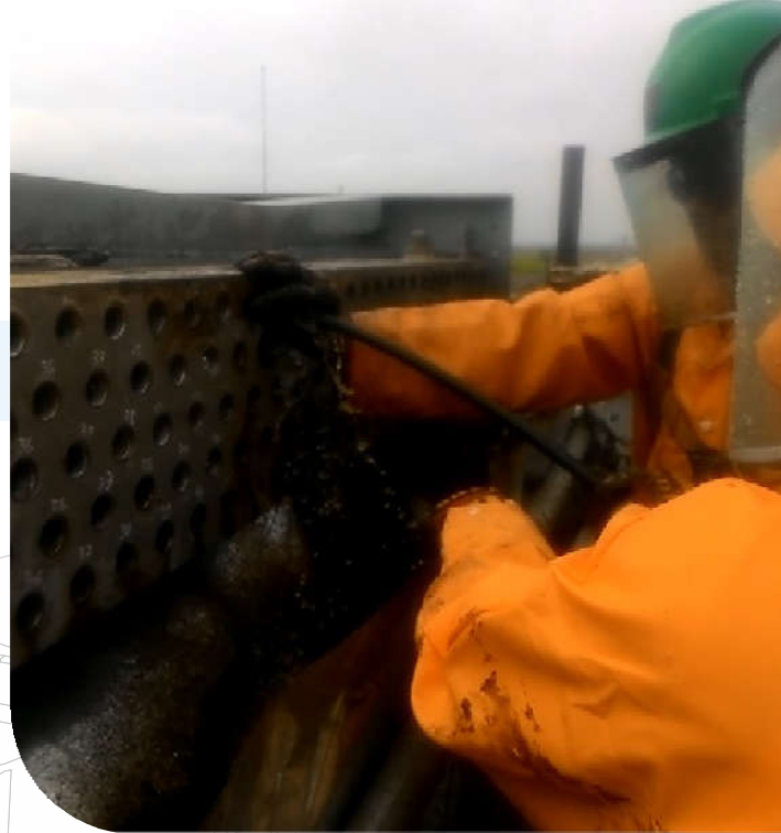
Mechanical Cleaning with Flexible Lance
