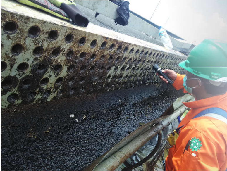
Inspection of Tube
