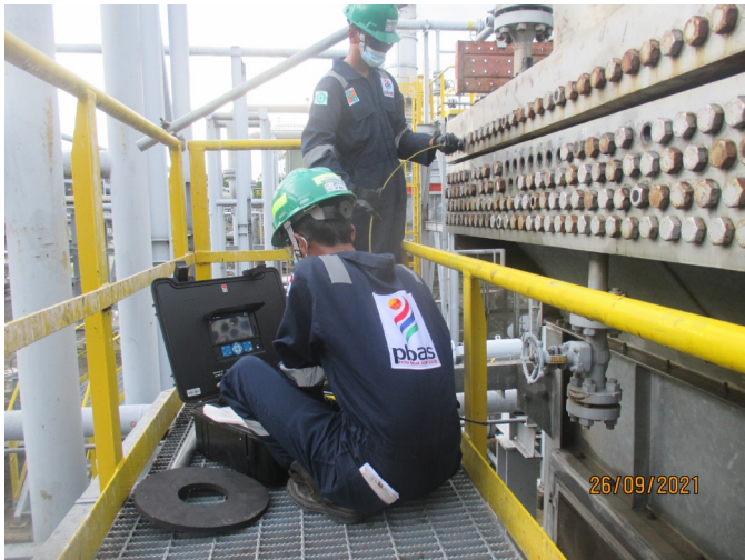
Tube Inspection with Borescope
