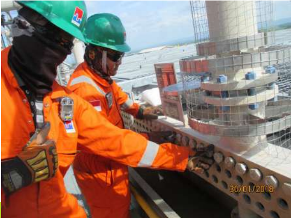
Inspection of Header Box
